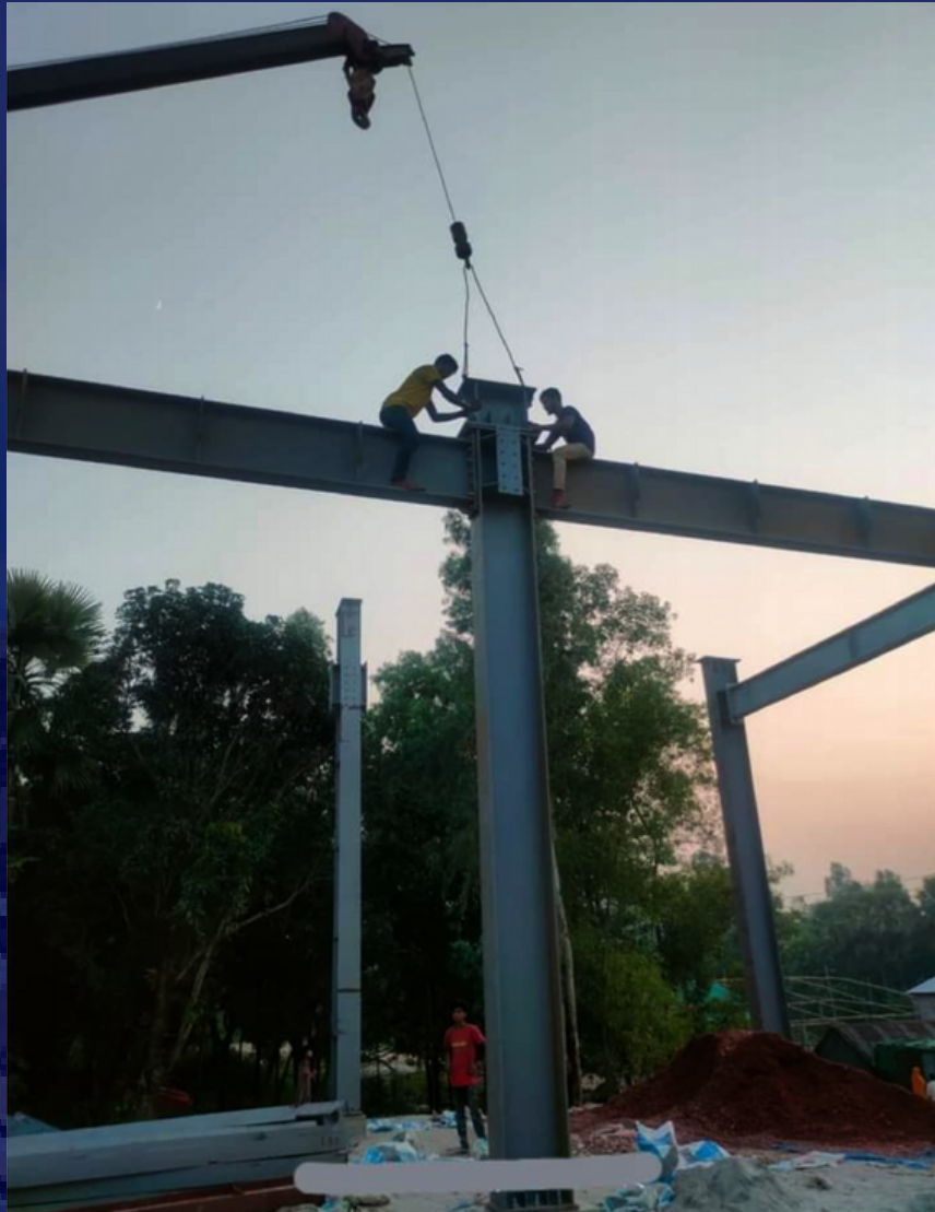
Factory Shed , Joint Builders, Nasirabad, CTG
