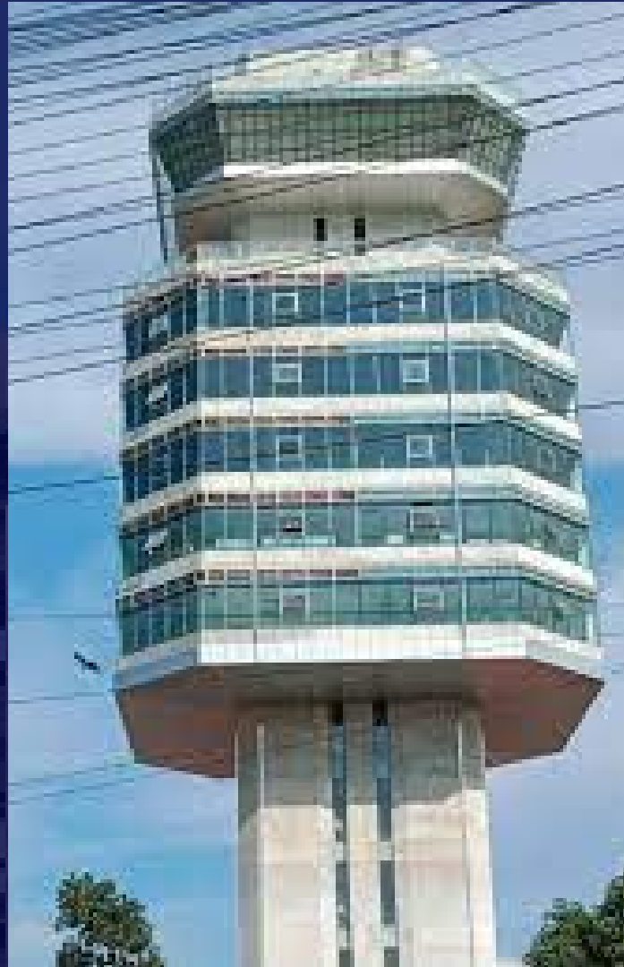
CTMS Tower( Watch tower) ,Chittagong Port
